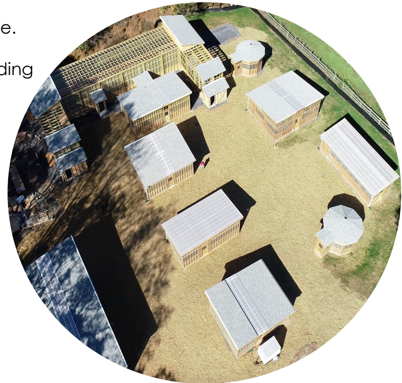
Aerial view of new facility outdoor enclosures
